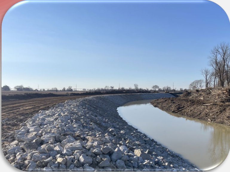
Ditch 19 Channel Cleanout
