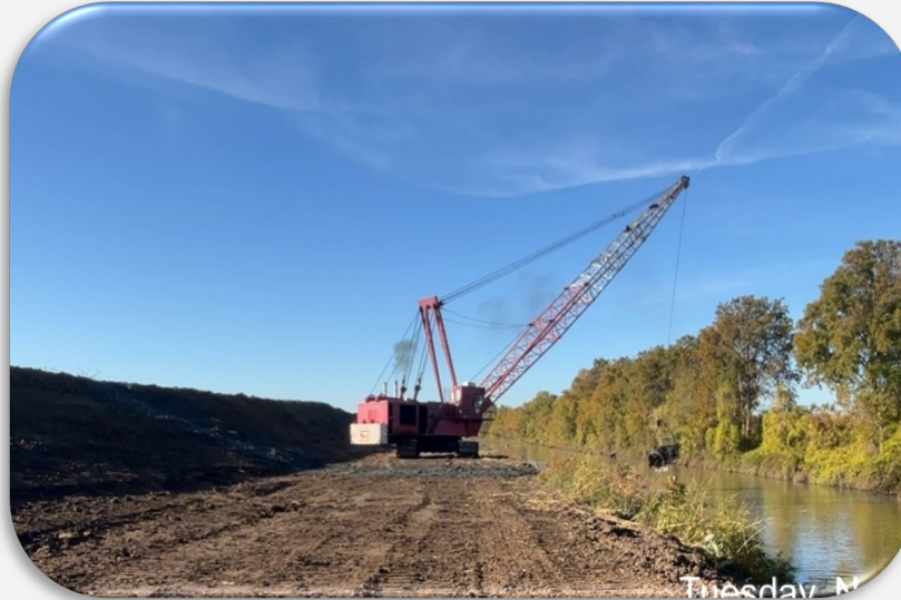
Belle Fountain Ditch Cleanout
