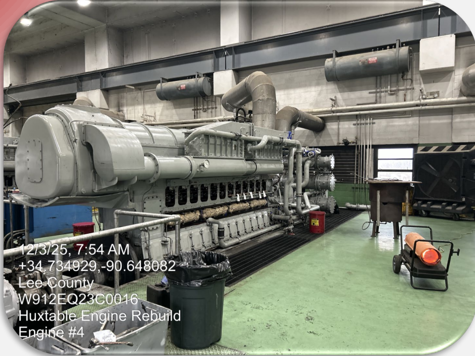
Huxtable Engine Rebuild
