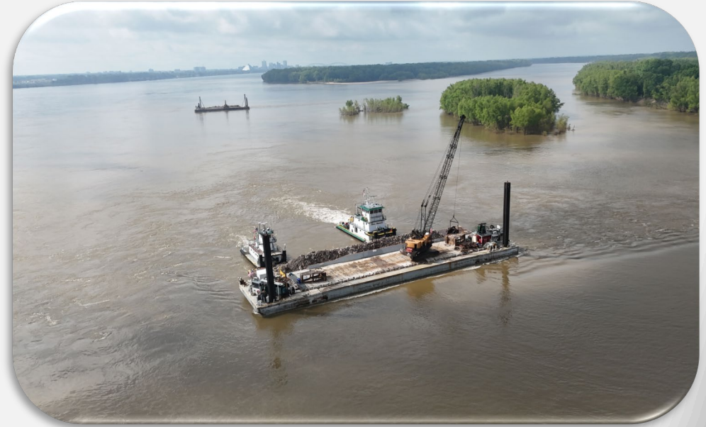
Sycamore Chute Dikes Stone Repairs
