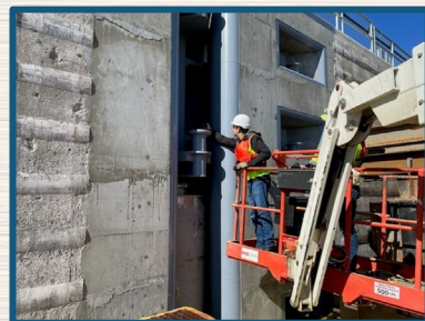
Lock 25 Phase 1 – Construction Complete
